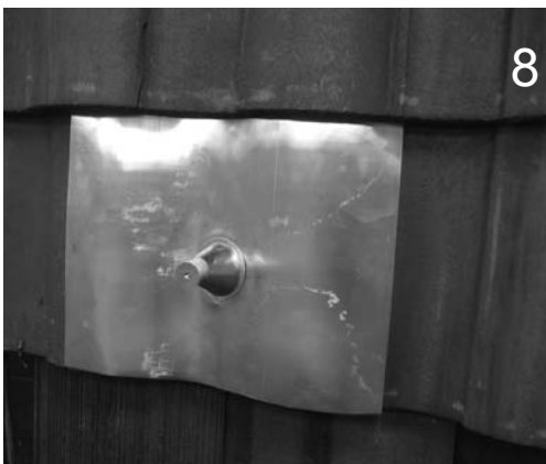
Place Aluminum Flashing into position over Post & bend to contour of tiles. Apply Sealant around cone to Post. Slide on EPDM Counter Flashing. Seal top of Post with 1 1/4" Sealing Washer.
