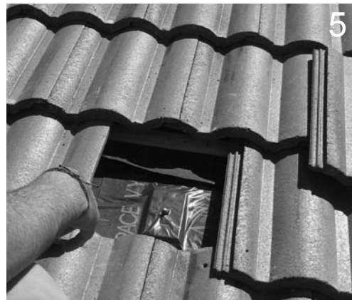
Carefully clean the building paper then install Peel and Stick Flashing over stud and up roof to lap under the next row of base paper flashing.
