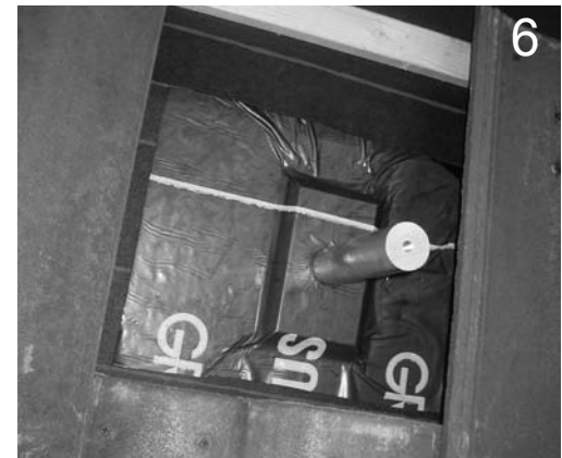
Take care to do a quality installation – see important notes *(below) and *(pg1). Firmly press Peel and Stick Flashing to Base and paper; work from center out removing any air pockets.
