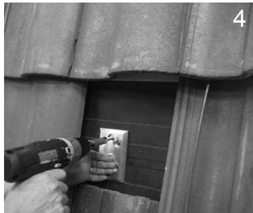
Drill 1/4" pilot hole. Place Machine Bolt under Base Plate in hex slot, threads pointing up. Lag Base Plate into Rafter on Marks.
