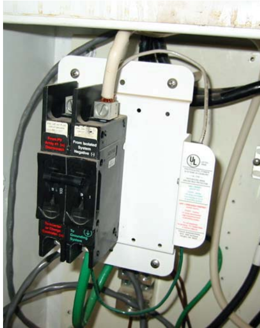
Figure 12. External Ground-Fault Protection Device
