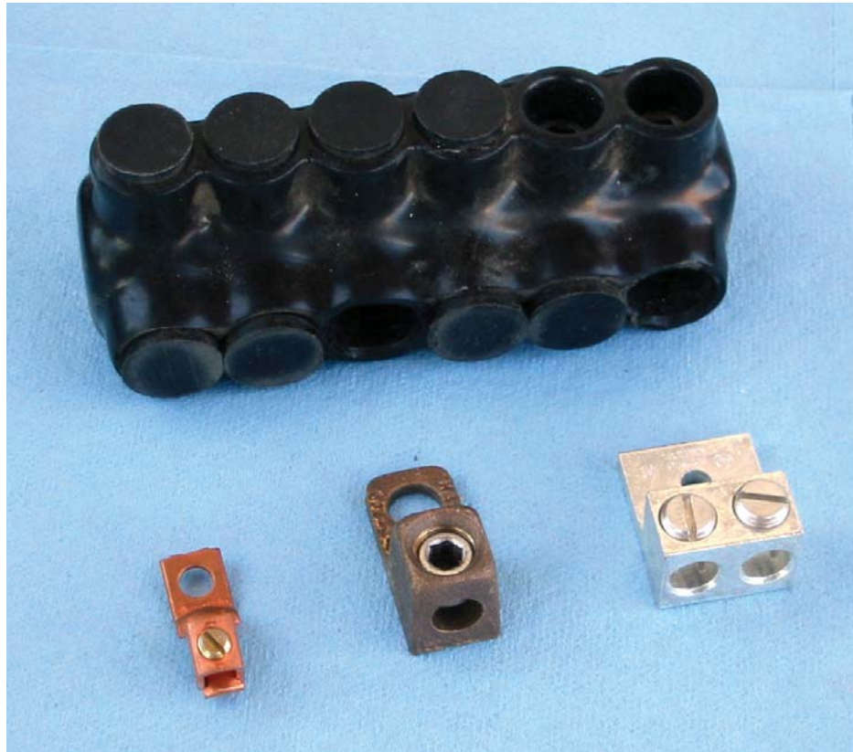
Figure 6. Listed Mechanical Terminals
