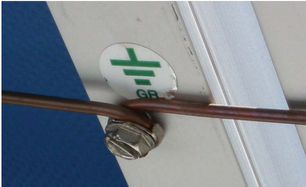
Figure G-3. Improper Module Grounding
