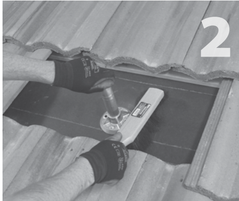
Clean away dust and debris around QBase.
