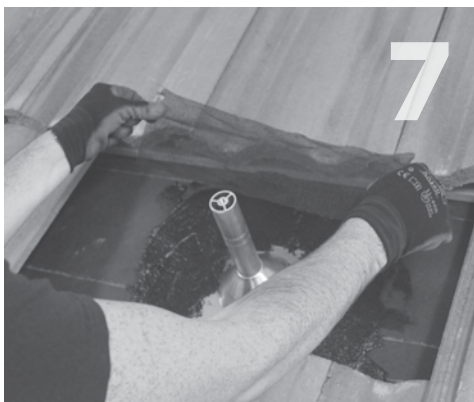
While cement is still wet apply 3 pieces of reinforcing fabric strips where felt paper and flashing meet – a 14" strip along the top, and a 10" strip along each side.
