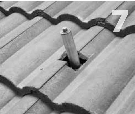
With a diamond blade on a grinder or skill-saw, cut tile to allow post to pass through. Place cut tile back in position. Insert post (item 3) and tighten into place.
