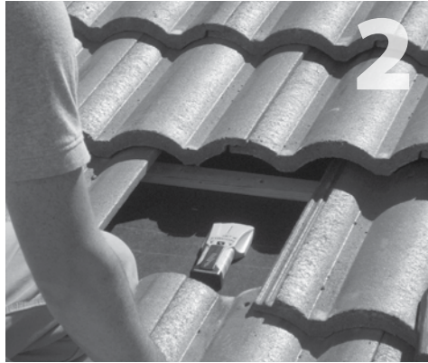
Locate and mark center of rafter. Clean felt paper with hand broom.
