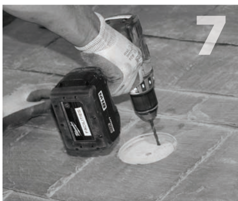
Using QBase (item 2) as a guide, align two clearance holes vertically with the center of the rafter. Mark the center of these 2 holes. Drill 7/32" pilot hole at each of the 2 marks. Hold drill square to rafter. Do not use QBase as a drill guide.
