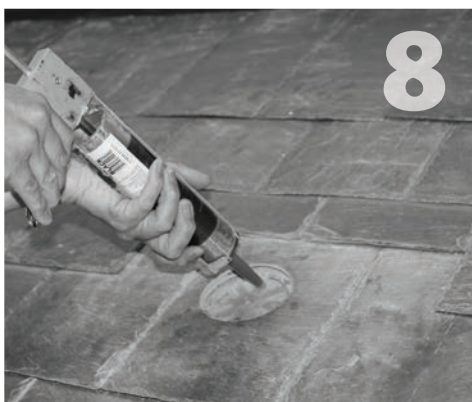
Fill pilot holes with sealant compatible with roofing material such as Chemlink M-1, Geogreen 4500, or Solar Seal 900.
