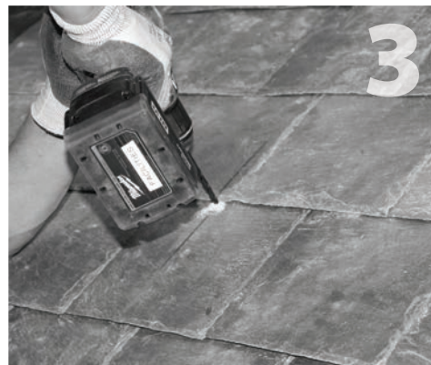
Using a masonry drill bit, drill a pilot hole at the center of the QBase location you marked in step 2. This drill bit should match the size of the guide bit of your hole saw.
