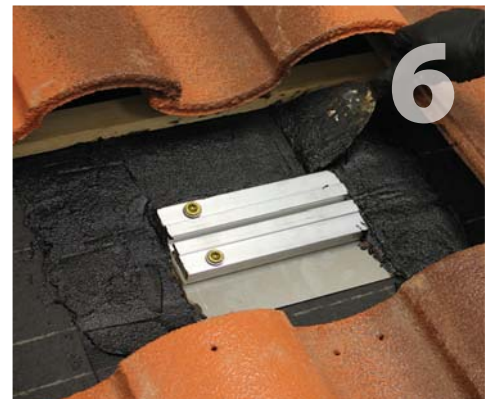
After first layer of cement is dry, apply second layer over fabric to finish waterproofing of sub-flashing.
