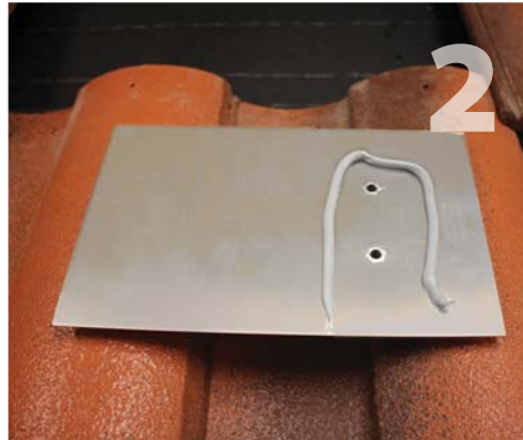
Apply a bead of sealant in the shape of an upside down U on the back side of the base mount around the lag holes. Bottom of U should point towards roof ridge
