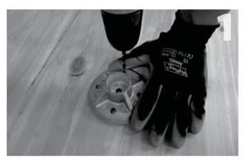
Locate the desired mount placement over a rafter (or custom wood blocking). Using the base as a template, mark the two penetration points with either a pen or light drilling. Use two opposing holes on the base plate, parallel to the structural member.
