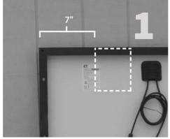
In a standard landscape array, the Enphase inverter bracket will be installed approximately 7" in from the edge of the module.
