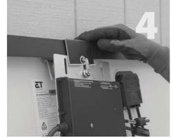
Slide the entire unit up under the bracket clamp, and then slightly to the left so that the cap screw holds everything together.
