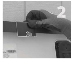
Place the bracket clamp over the edge of the module frame.
