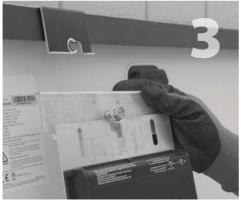
With the cap screw threaded into the channel on the bracket, slide the Enphase inverter on top of the bracket with the cap screw in the middle channel on the inverter.
