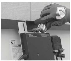
Tighten the cap screw with a half-inch socket and torque wrench. Torque to 15 foot-pounds.
