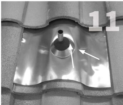
Slide the appropriately cut collar over the conduit all the way down to the flashing.
