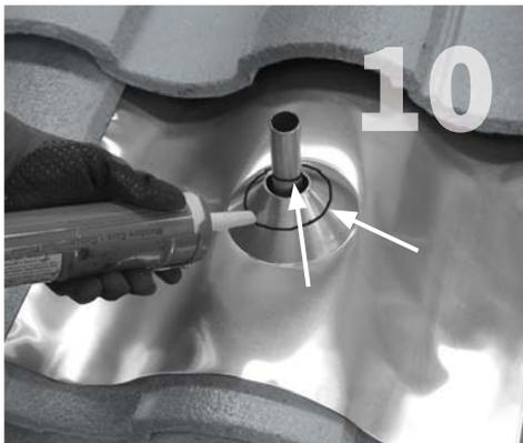
Apply a bead of sealant compatible with the EPDM rubber to both the flashing and the conduit in the location of the EPDM collars final position.
