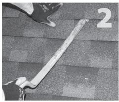
Carefully lift composition roof shingle with roofing bar, just above placement of mount. Remove nails as required. See "Proper Flashing Placement" on next page.
