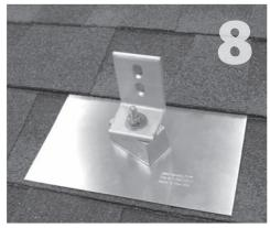
Using the rack kit hardware, secure the racking (L-foot) to the mount using torque specs from racking manufacturer. If racking manufacturer does not specify torque setting, tighten to 13 ft.-lbs.
