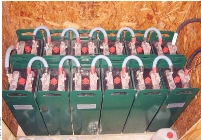
Twelve 2 V IBE batteries in individual steel cases, wired as a single string for 24 V.
