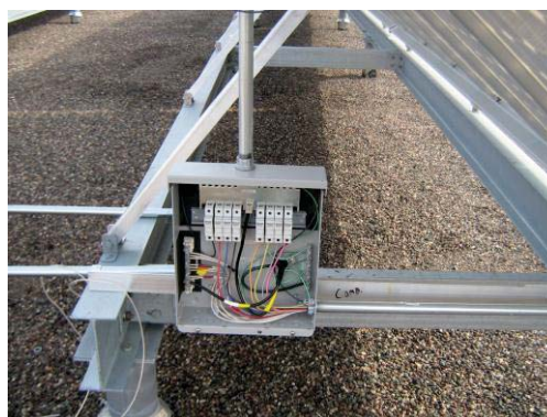
Box lug and screw placement for fuse holder configuration
