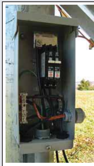
Installation photo courtesy of APRS World
