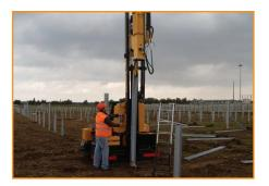
This foundation method requires analysis to understand the bearing capacity and corrosivity of the soil (performed by a Geotechnical Engineer). From an installation standpoint, specialized equipment and operators are required to install these types of foundations which increases the overall system costs. Additionally, this option does not utilize a helical blade or screw, which means that it will have a lower resistance to uplift forces. This necessitates deeper foundations.
