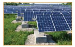
This is a common foundation method especially for brownfield sites, such as landfills, where there is a cap layer that cannot be penetrated. Ballast foundations can be either cast-in-place or pre-cast depending on project requirements and shipping costs.
