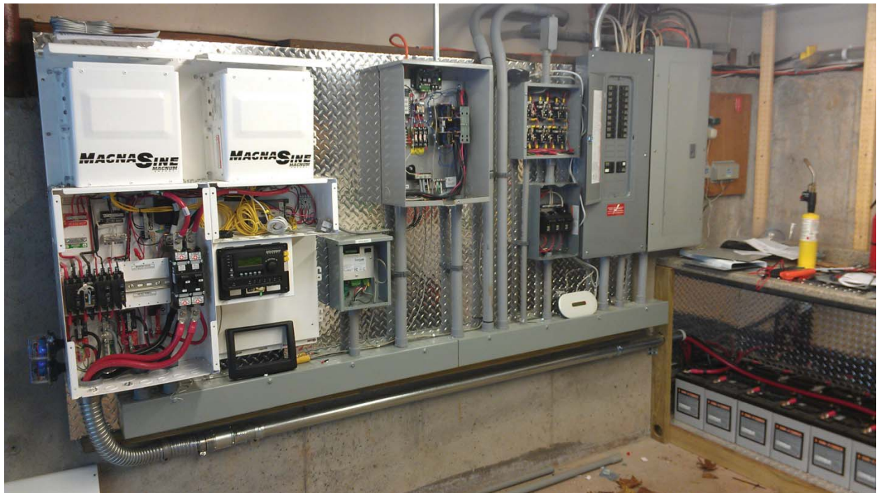
The Power Room of an AC Coupled System with Enphase Microinverters, Courtesy of Magnum Energy
