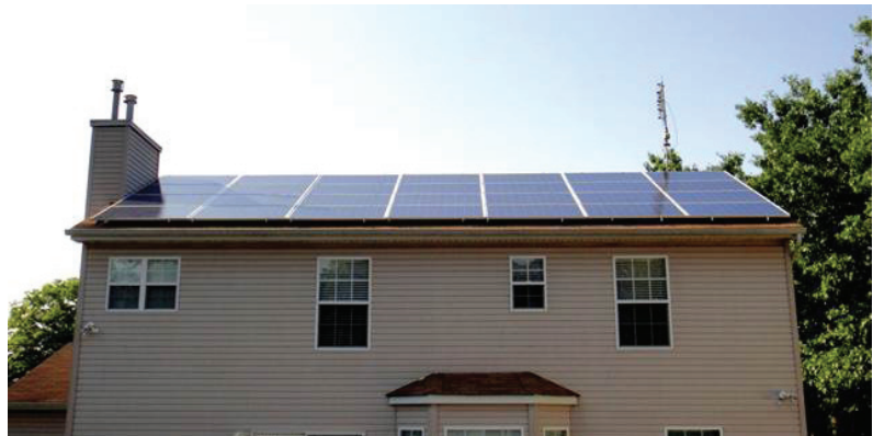
Figure 2: SolarEdge allows for full roof utilization despite shading elements (here: chimney). Full roof utilization can only work if the MPPT range of the module-level device goes low enough to prevent module bypass diodes from being activated.
