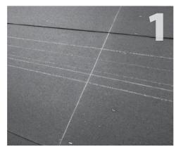
Layout your array out over the roofing paper using Align QBase vertical holes over center rafter mark a chalk line to mark rafter centers and the rail location center.
