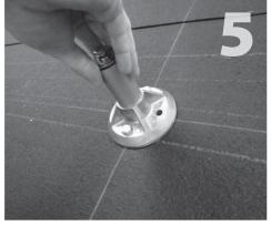
Secure post (item 2) to QBase turning post onto Allow roofing to proceed to the point that the captive base plate bolt.
