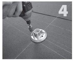
Fill pilot holes with sealant compatible with roofing material. Seat grade 8 cap screw (item 3) through bottom of QBase (item 1). Place QBase over drilled holes and secure lags (item 4) in place, to a solid, snug fit.
