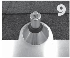
Apply sealant where post and flashing meet. Install EPDM counter flashing collar (item 6). Seal post with hardware (item 7-10) if not installing racking right away.
