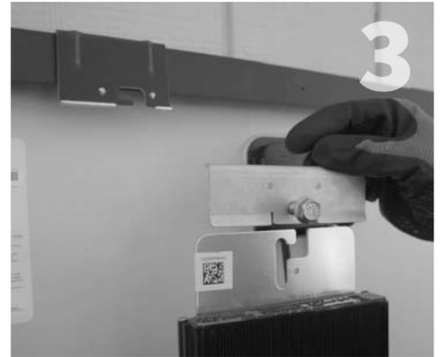
With the cap screw threaded into the bracket, slide the cap screw into the slot on the module level electronic mounting bracket with the bracket behind the module level electronic mounting bracket.
