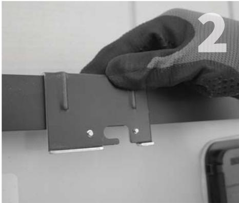
Place the bracket clamp over the edge of the module frame.
