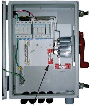
Step 4: Reinstall Positive block
