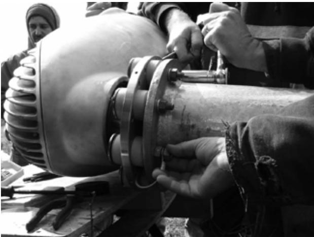
Fig. 13 Grounding turbine to tower
